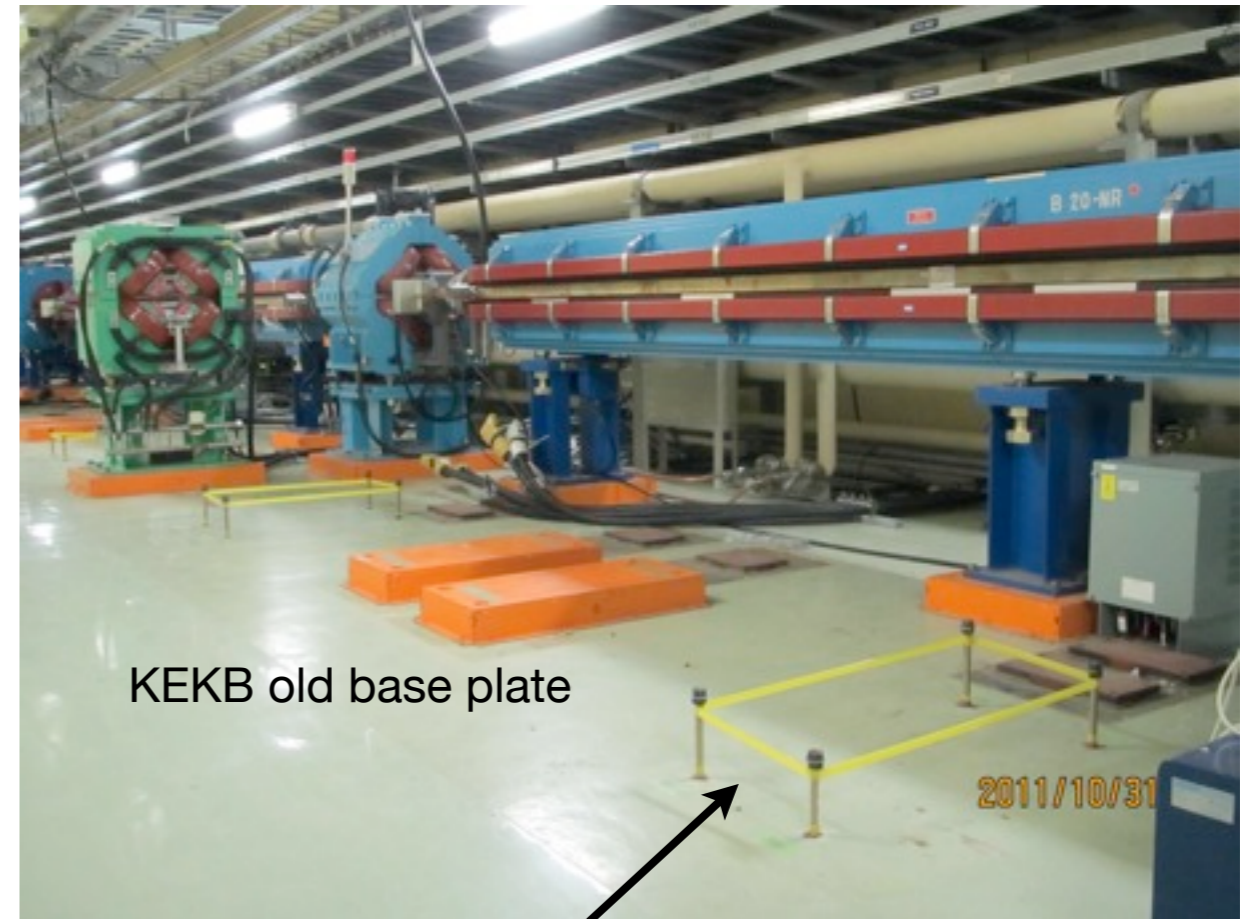
Anchor bolt for base plate (new 4.2 m bending magnet)
