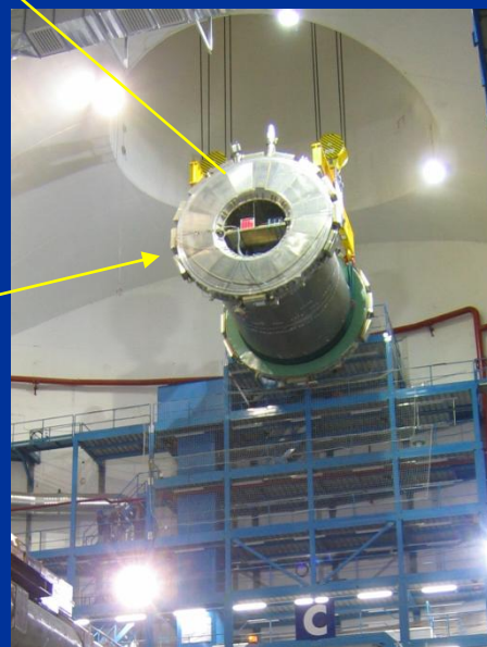
Liquid argon barrel calorimeter cryostat during lowering in the pit
