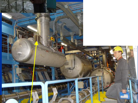
Phase separator cryostat for Toroids
