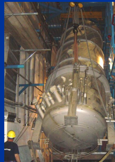
15000 liter nitrogen phase separator
