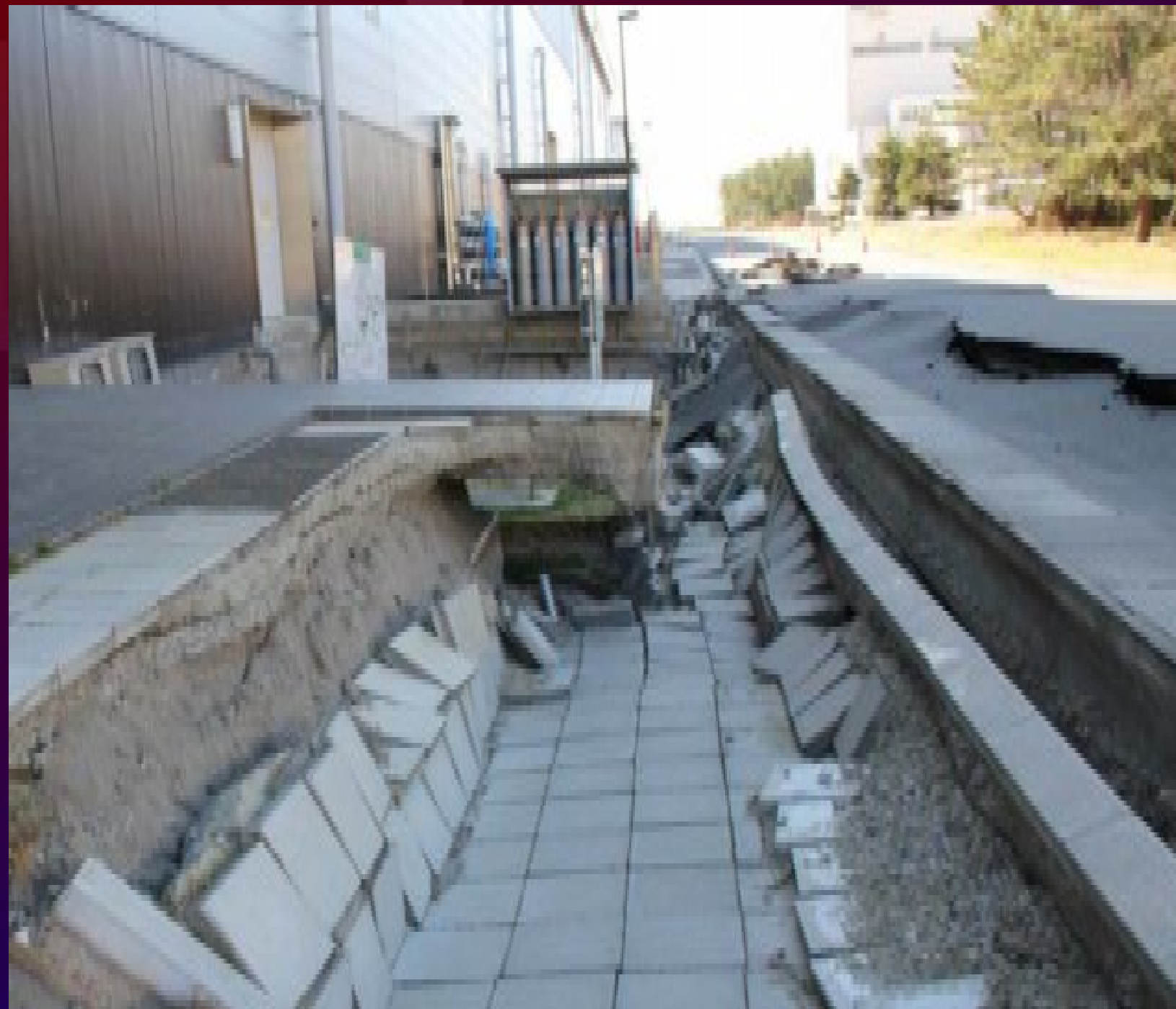
LINAC building entrance
