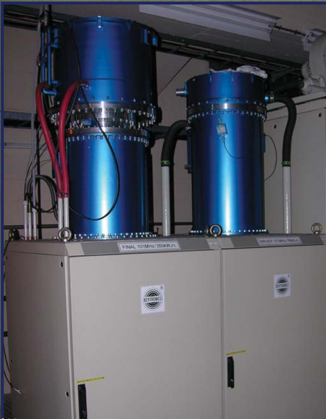
CERN Linac3: 100 MHz, 350 kW 50 kW Driver: TH345, Final: RS 2054 SK
