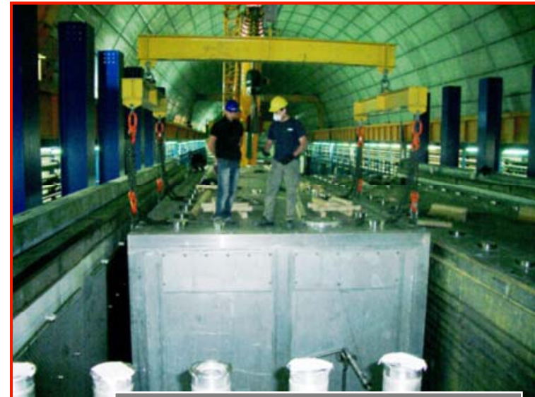
Almost in place
