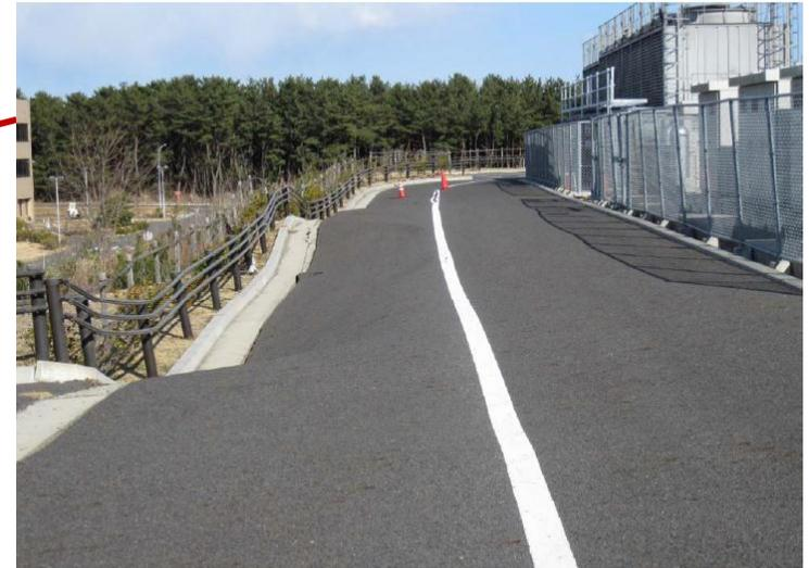
Wave road. Bump in the middle. Both sides of the bump were sinking. Capacitor bank and transformers
