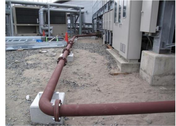
Damaged water pipes were replaced to enable cooling.
