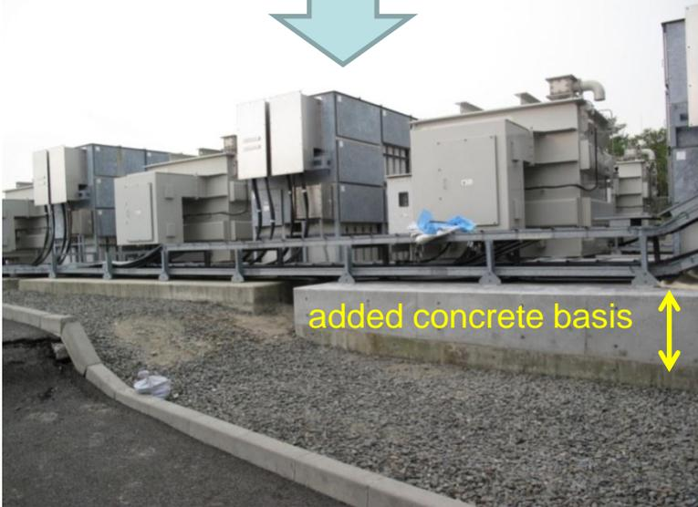
Tilted capacitors were straightened after re-leveling the bases.
