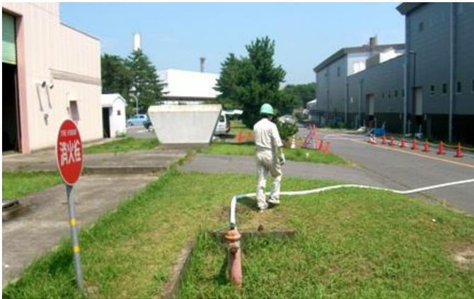
We are getting water from an outside fire-hydrant, as original cooling water system has not yet been fixed.
