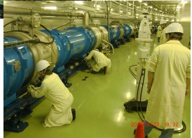
Realignment work of electromagnets (above) and superconducting magnets (below) is progressing smoothly. We also try to improve cooling power.
