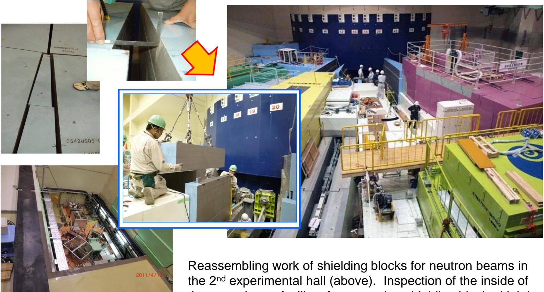
Reassembling work of shielding blocks for neutron beams in the 2<sup>nd</sup> experimental hall (above). Inspection of the inside of the muon beam facility after removing shielding blocks (right). This area does not have any serious damage.
