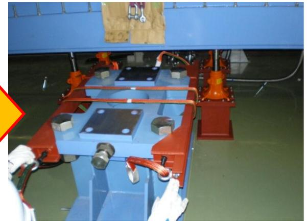
Pulling out the stage to put new longer height-adjust screws
