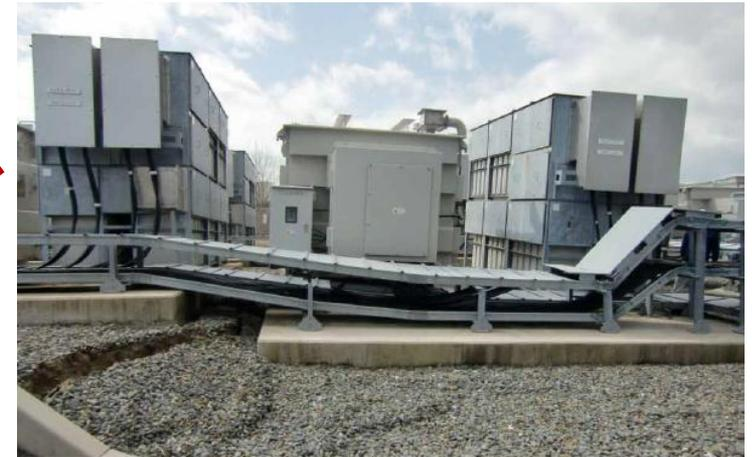
Capacitor bank and transformers were tilted. Cables were distorted with heavy weight on them.
