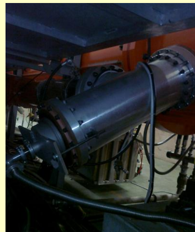
RF feeder loop – Tank 2 Bell installed – Rotary Pump
