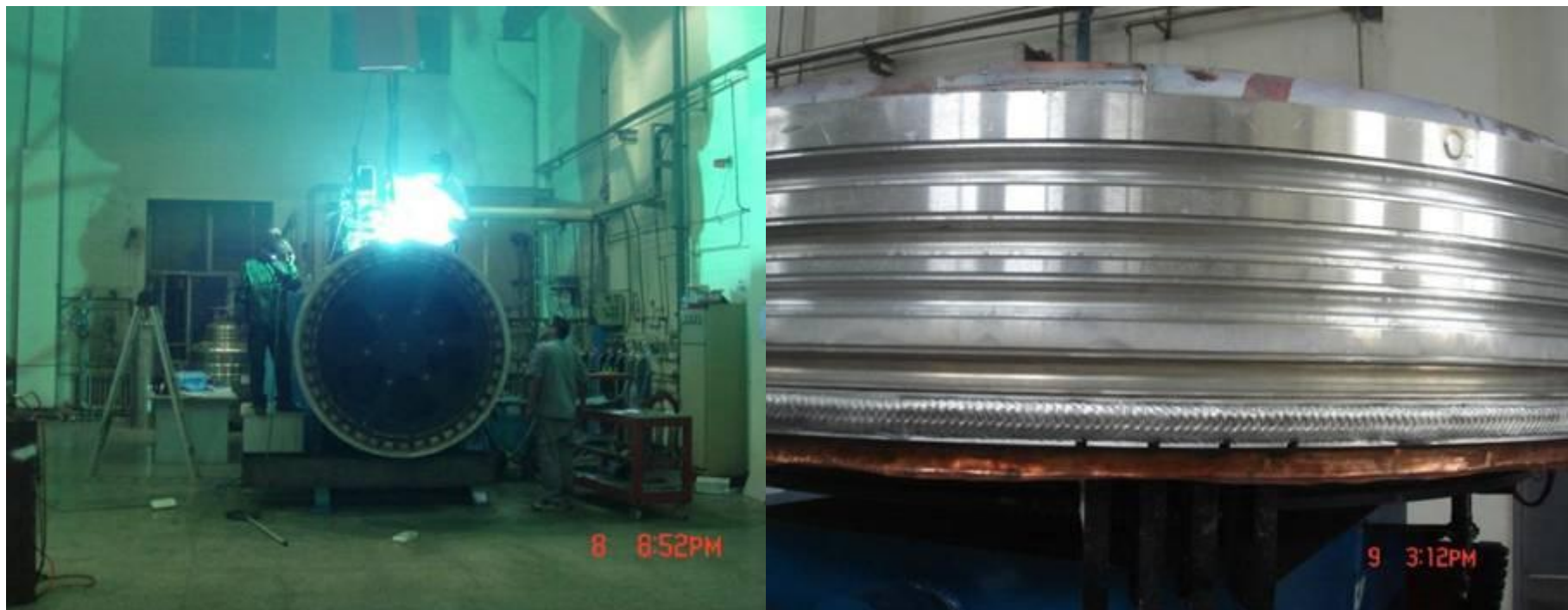
Cover plate welding at HIT in early August 2011
