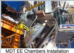
During the 2011 shutdown period, 26 MDT chambers were installed on side C (completed) and 2 MDT chambers were installed on side A. This upgrade will improve the muon momentum resolution and acceptance in the corresponding region of the Muon Spectrometer for the high pT physics analysis.
