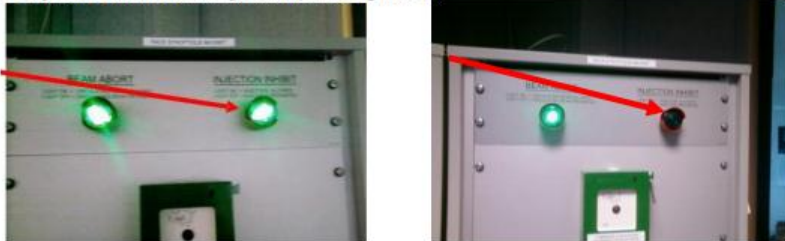
Figure 1. The injection inhibit button. The left picture show the condition where the pixel HV must be OFF (Injection enabled) while the right picture show the condition where the Pixel HV can be turned ON (Injection inhibited).
