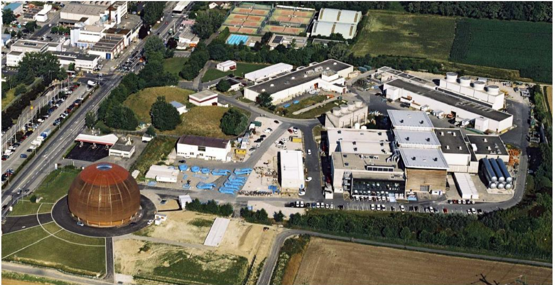
(Across the street from the CERN main entrance)
