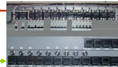
Temperature and current of heaters controllers
