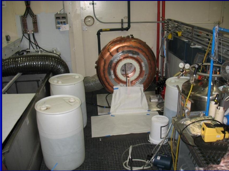
EP setup in plating shop at LBNL
