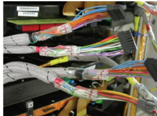
repaired cables with shrinkage tube
