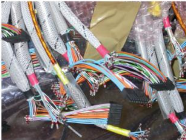
cables after Y-type crimping
