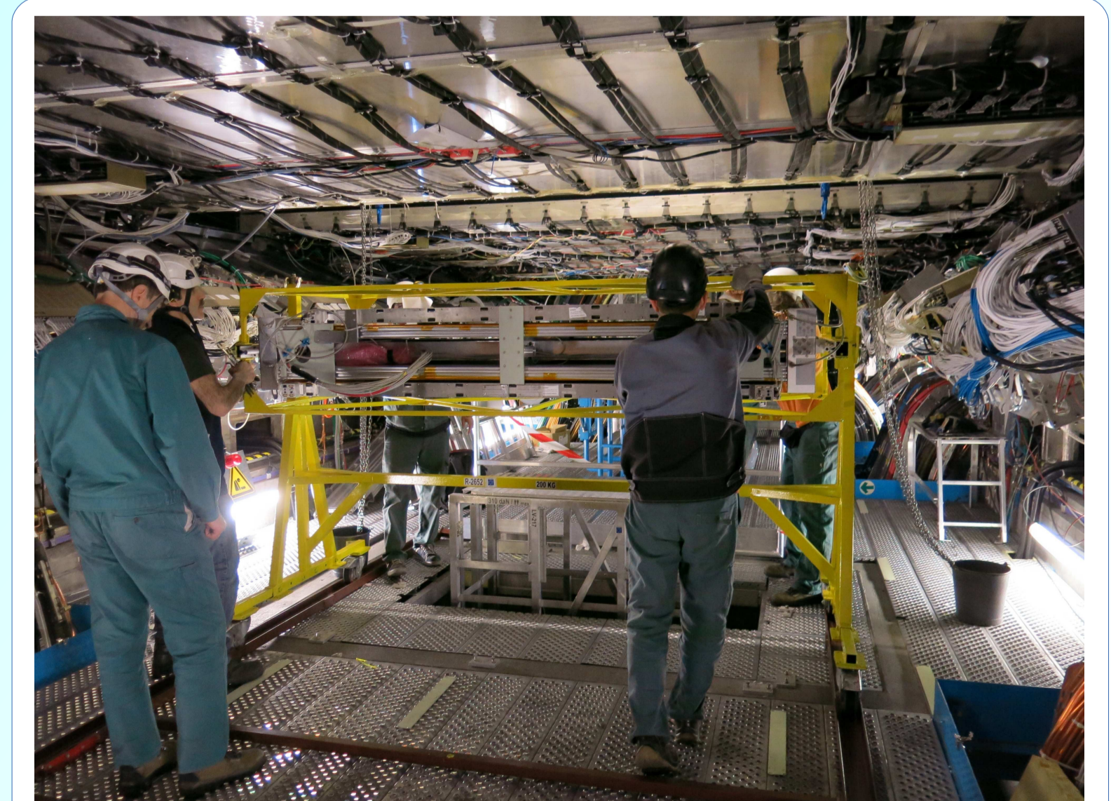
Installation of BME A side chamber in the ATLAS cavern
