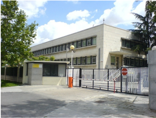
Main Offices (Moncloa)
