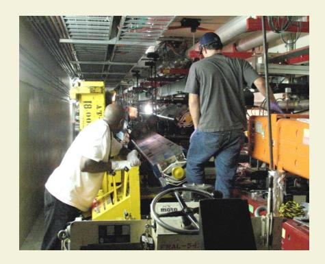
Replacing a primary beam 3 meter dipole. Ceramic isolator water leak.
