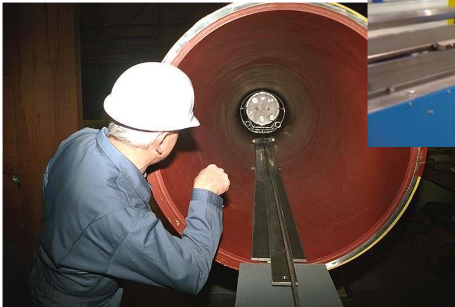
Pulling through sliding on vacuum vessel
