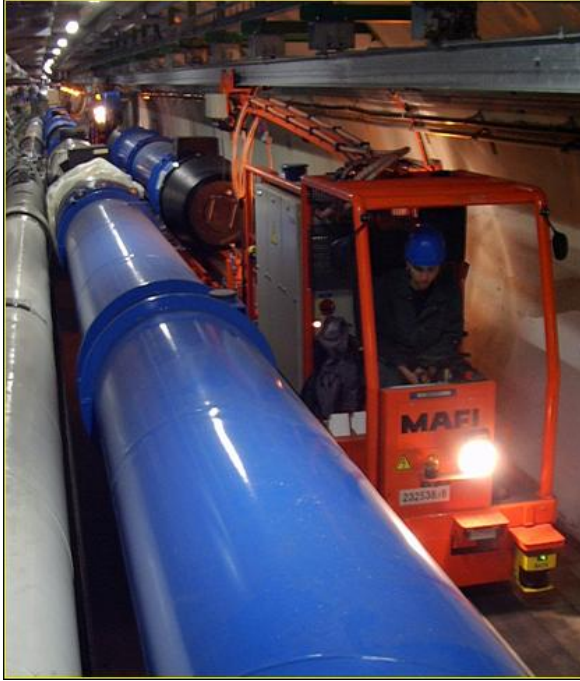
Figure 3: Transport of magnets in the LHC tunnel.
