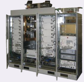
In tunnel alcoves
