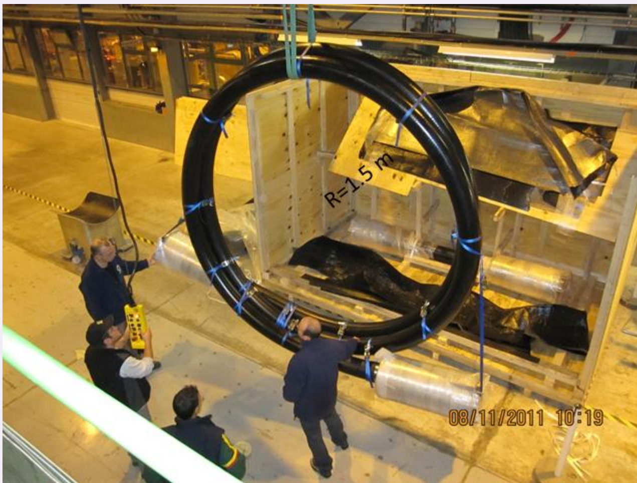
20-m Long Nexans Transfer Line
