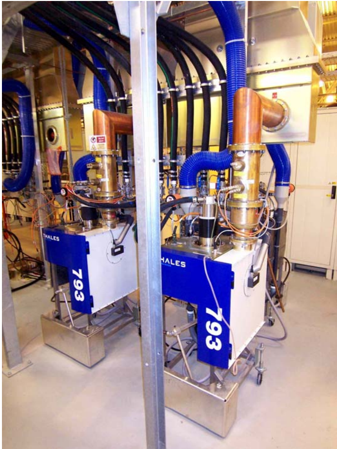
Diamond TH793 IOTs 450-850 MHz 80 kW cw
