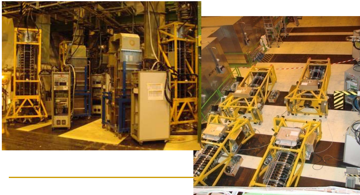
Klystrons in horizontal position in UX45
