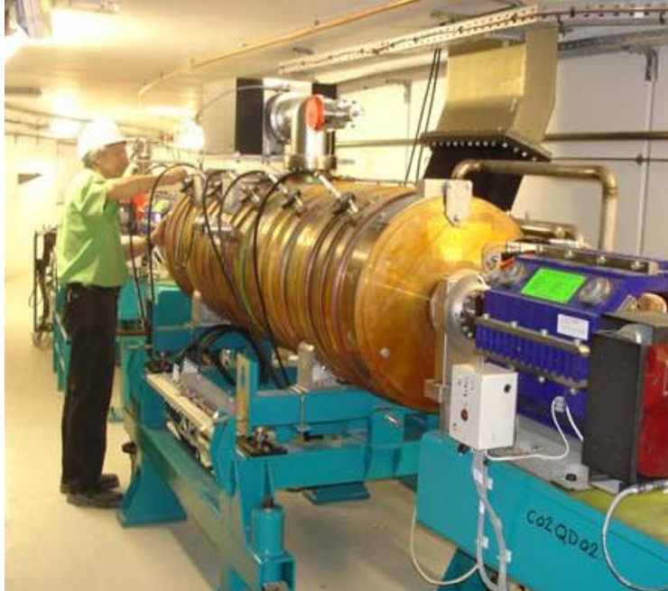
5-cell copper cavity of the LEP type in the SOLEIL Booster
