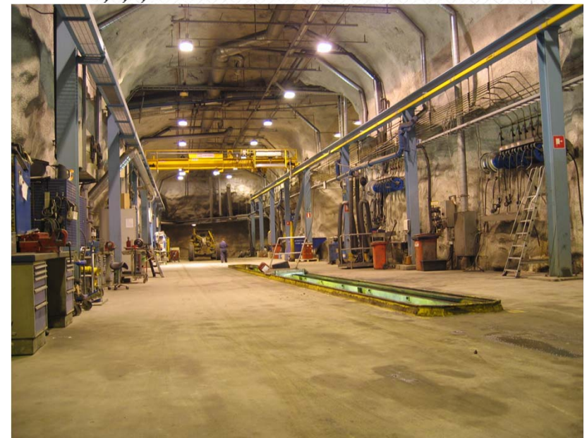
Shotcrete lining at -1430m in the maintenance hall in Pyhäsalmi, Finland)
