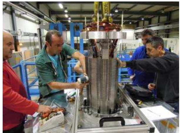
Fig. 3: A view of the final stage of collaring.
