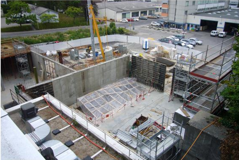
Top-view construction site: 10 July
