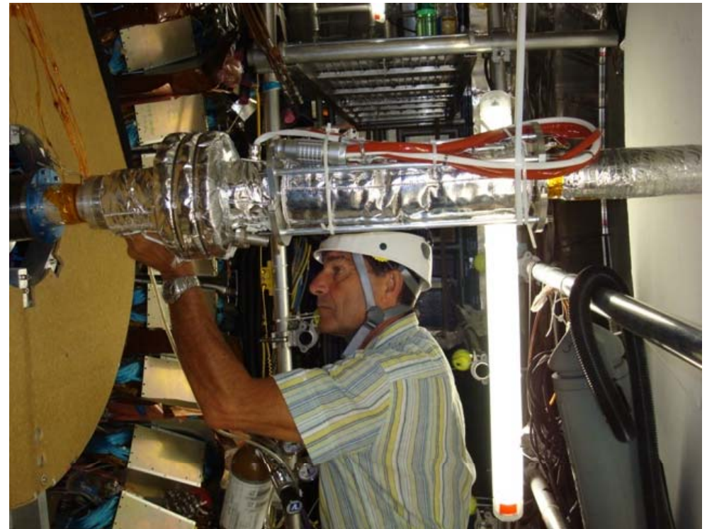
Connection of the ID section to the LAr EC beam pipe section
