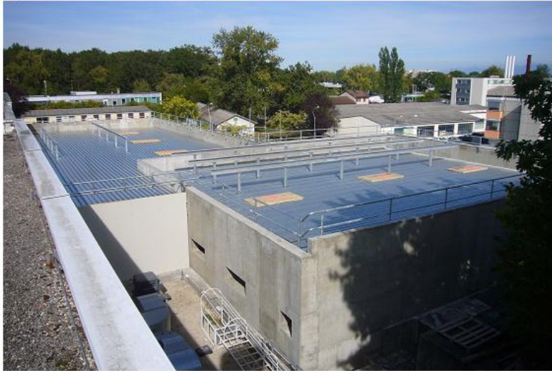
Top-view construction site: 20 September
