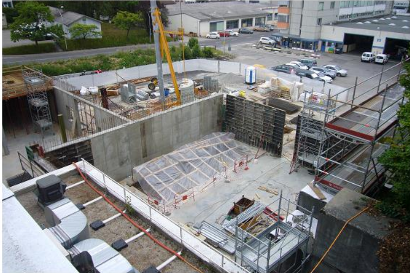
Top-view construction site: 10 July
