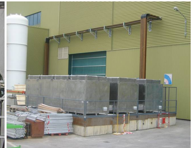
Dump resistors connected
