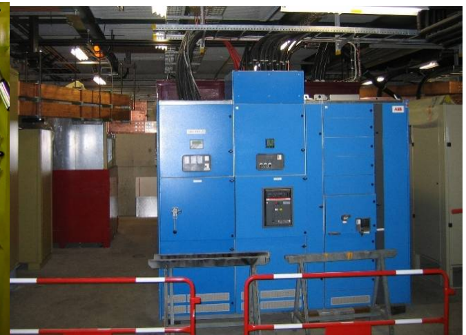
20 kA power converter tested
