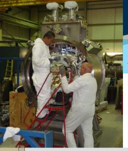
Installation of the He turret pipework
