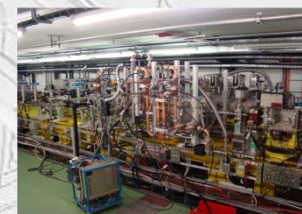
Final assembly of the AS vacuum tank.
