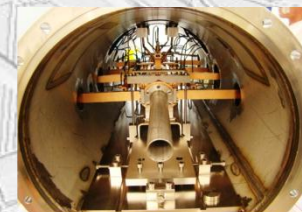
Installation of Input and Output waveguides
