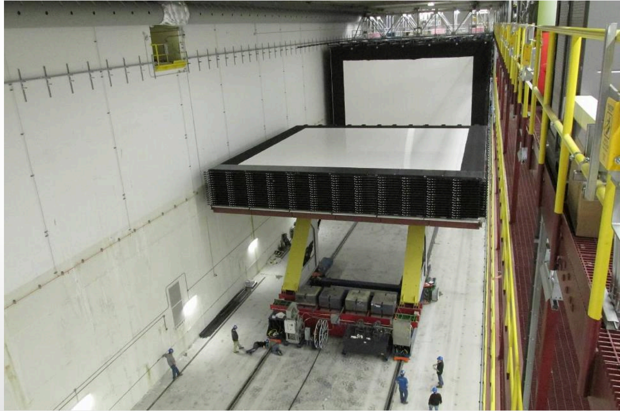
A completed detector block being moved into place at the Far Detector hall.
