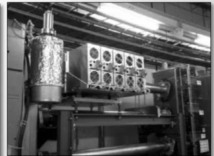
... installed in PSB ring 4
