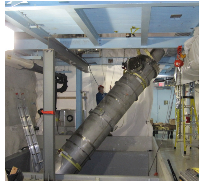
Parts of LAB processing system arriving on site
