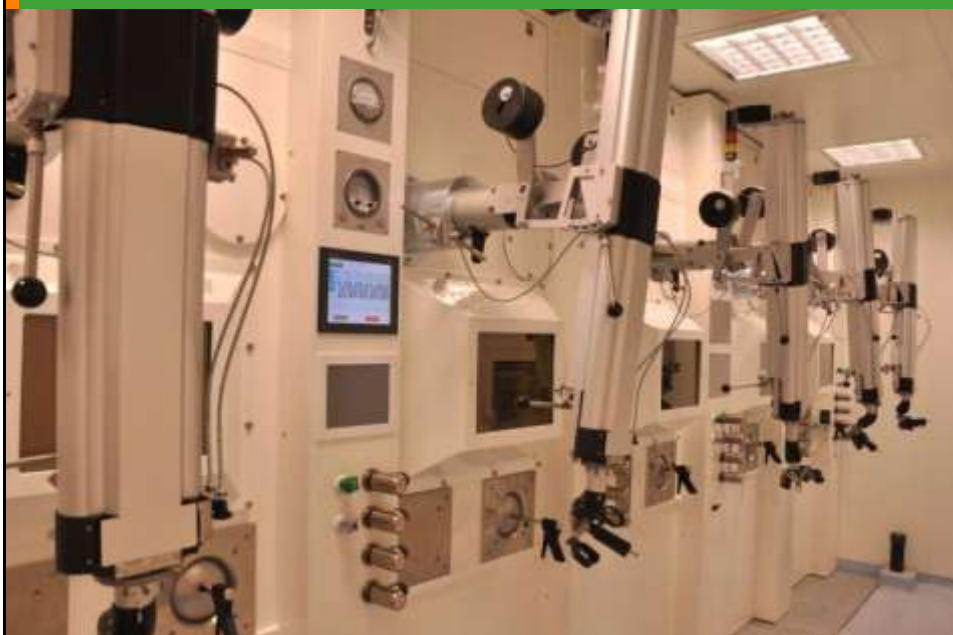
The Nantes cyclotron in September 2010
