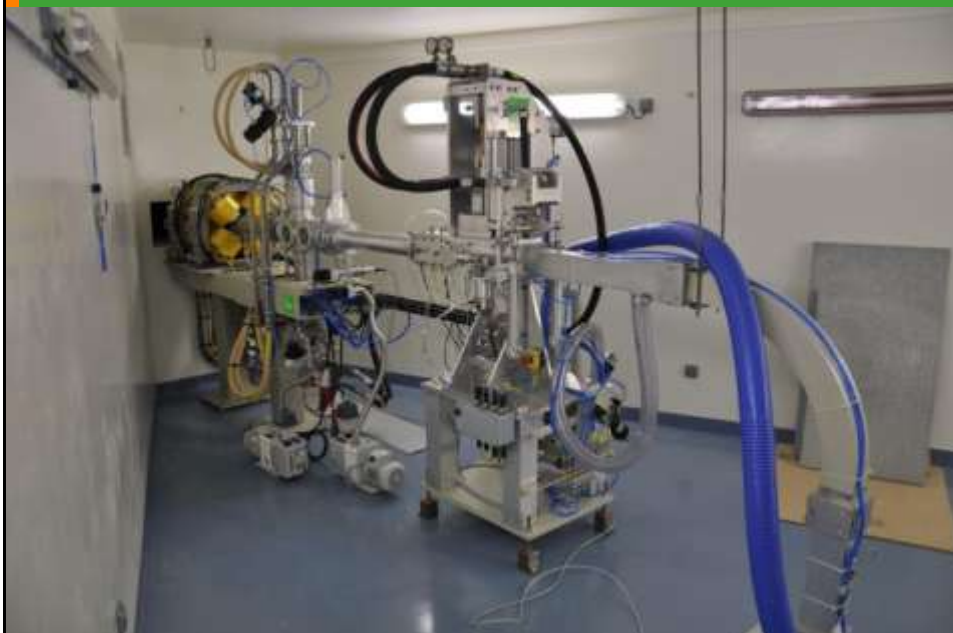
The Nantes cyclotron in September 2010
