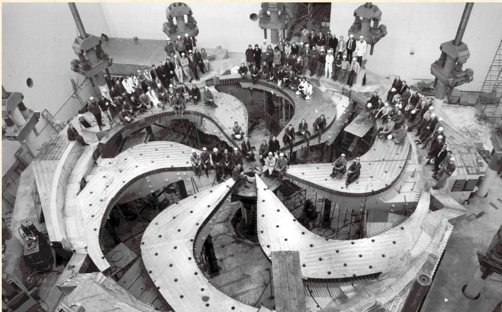
Lower half of the Main Magnet poles
