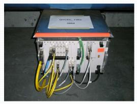
• More than 800 instrumentation crates are installed, connected and tested underground. They house electronic cards for the temperature (TT), pressure (PT) and liquid helium level (LT) measurements, supply electrical power to the cryogenic heaters (EH) and read the digital valve status
