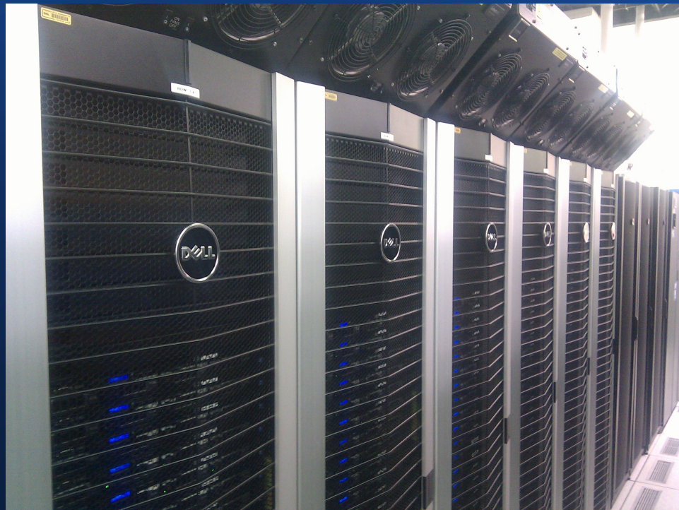
New RHIC Dell R410 servers with Liebert XD Overhead Cooling
