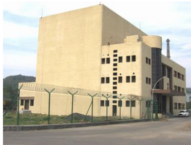
AHWR Critical Facility
