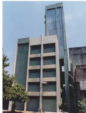
Building housing ITL
