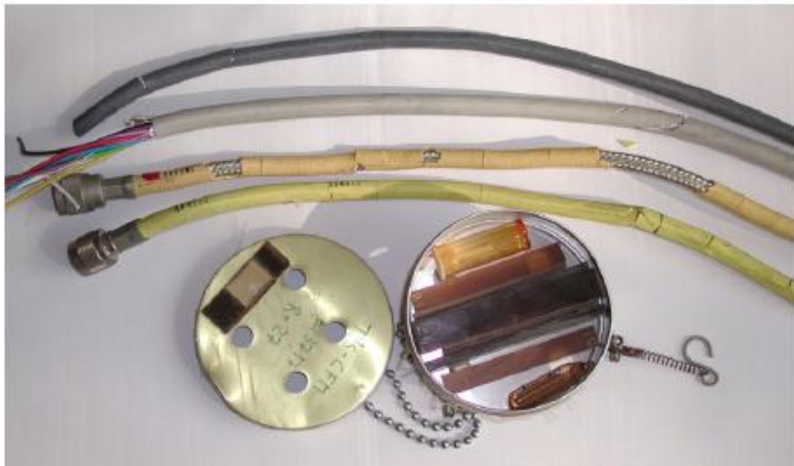
Fig. 17: some coaxial and control cables damaged by the radiation in LEP. Also seen on the picture is a metallic box containing samples of magnet insulating resins and dosimeters.
