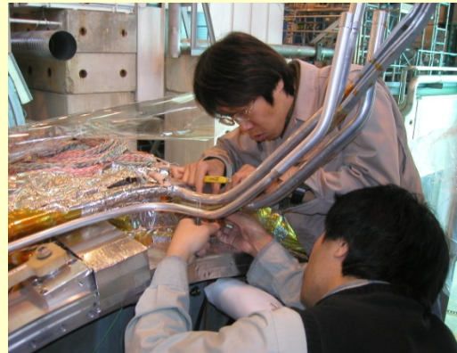
Connection works, cooldown and test (2004.2-9)
