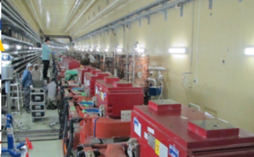
ARES cavities moved from HER to LER, and wiggler magnets for HER installed in D5 Oho straight section.
