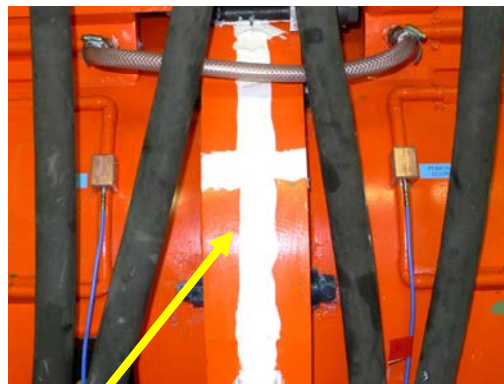
Resin poured and polymerised in situ (TS-MME)
