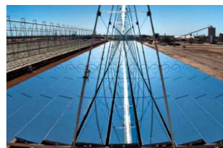
Thermal solar components (reflectors, receptor tube)
