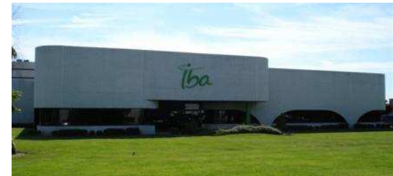
The IBA Long Island test facility
