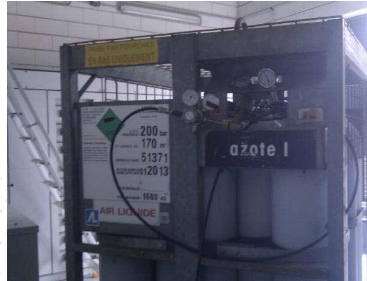
Technical shutdown of August: Installation of 18 cylinders on the main circuit allows us a 2-hours autonomy
