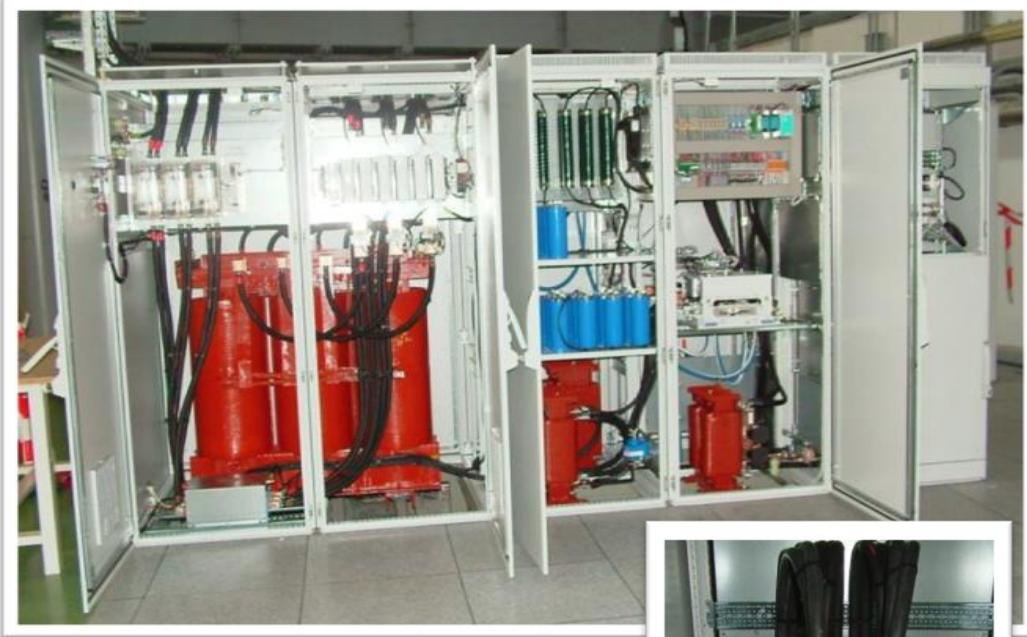
A new dipole storage ring power-supply (580A / 610V +/- 10ppm), has been in-house developed. Switching between power supplies takes less than 5 minutes
