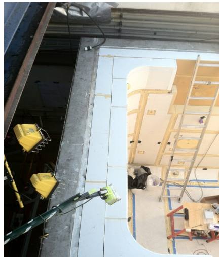
Top View of Two Layers Foam
