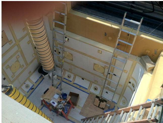
Two layers of foam (0.4 m)
