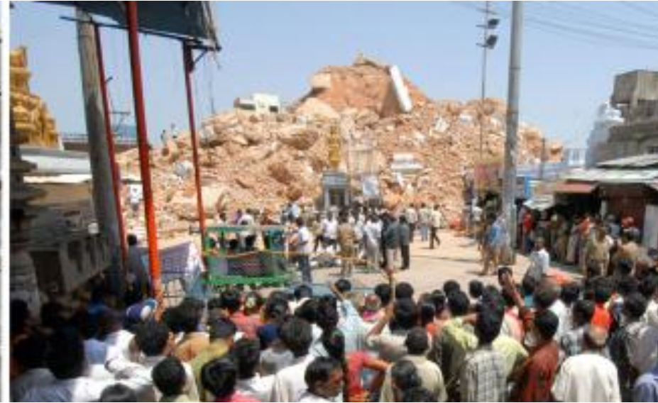
500-year-old Srikalahasti temple in Andhra Pradesh collapsed in 2010 – Foundations were only 45cm thick.
