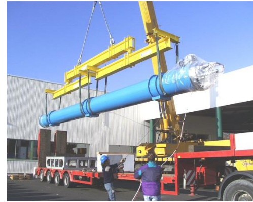
A 15m truck unloading a 27 tons LHC dipole
