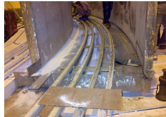
Cryostat pedestal ring- bottom plate (180 mm) & side plates (120 & 80 mm) are being welded together
